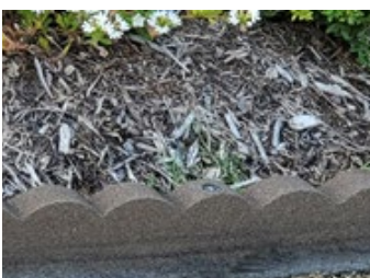
Scalloped concrete borders are prohibited.
