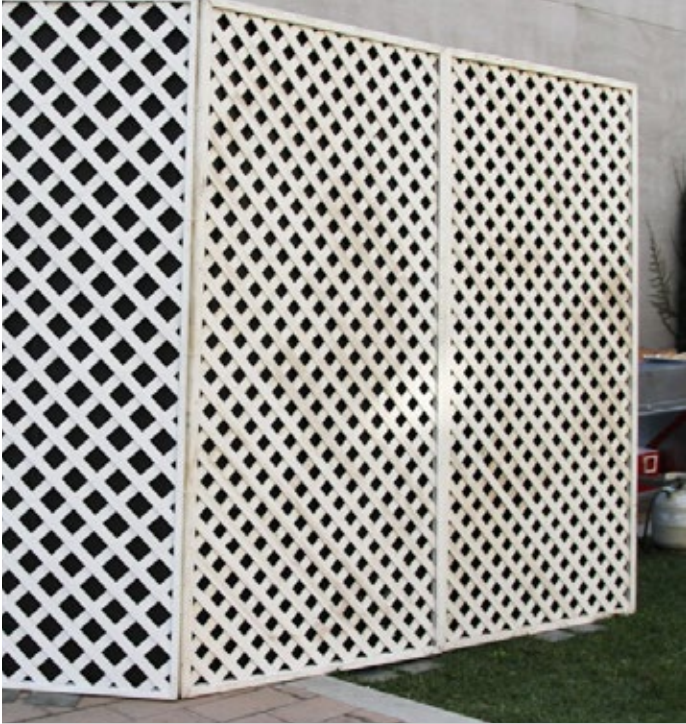
Plastic lattice is not acceptable.
