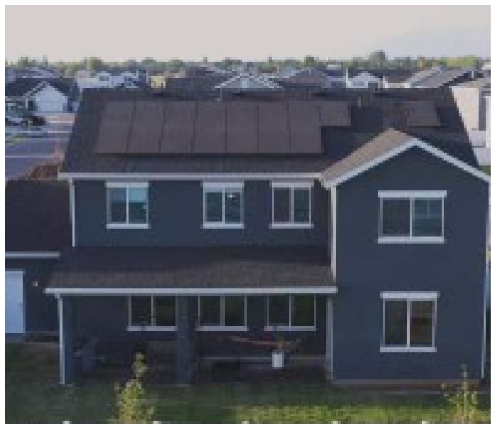
Solar Panels are permitted on the home's rear roof line.
