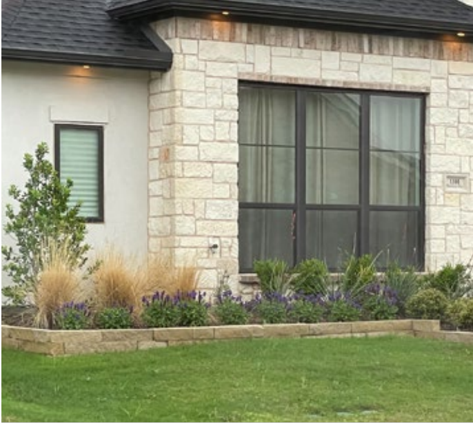
Eave lighting is appropriately spaced with the correct level of brightness, and is in the appropriate range of color temperature.
