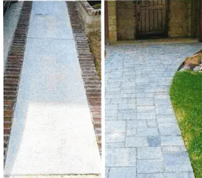
A paver edge to a concrete walk is permitted. Stone pavers are allowed as a concrete sidewalk replacement.
