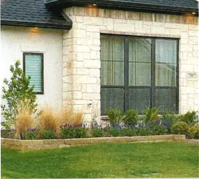
Eave lighting is appropriately spaced with the correct level of brightness, and is in the appropriate range of color temperature.
