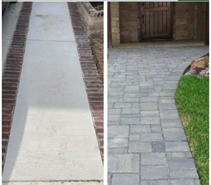
A paver edge to a concrete walk is permitted. Stone pavers are allowed as a concrete sidewalk replacement.
