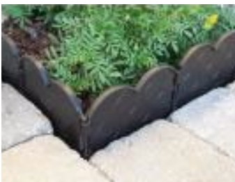
Scalloped concrete borders are prohibited.
