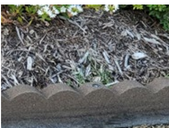
Scalloped concrete borders are prohibited.
